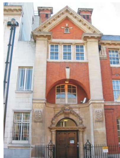
County Hall detail
