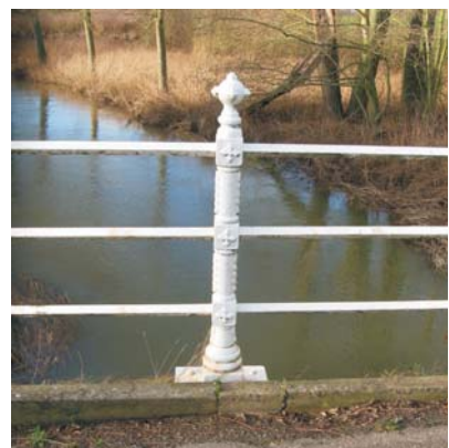
Howe Street Bridge detail
